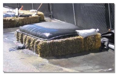
**Photograph DW-1.** A relatively small dewatering operation using straw bales and a dewatering bag.
